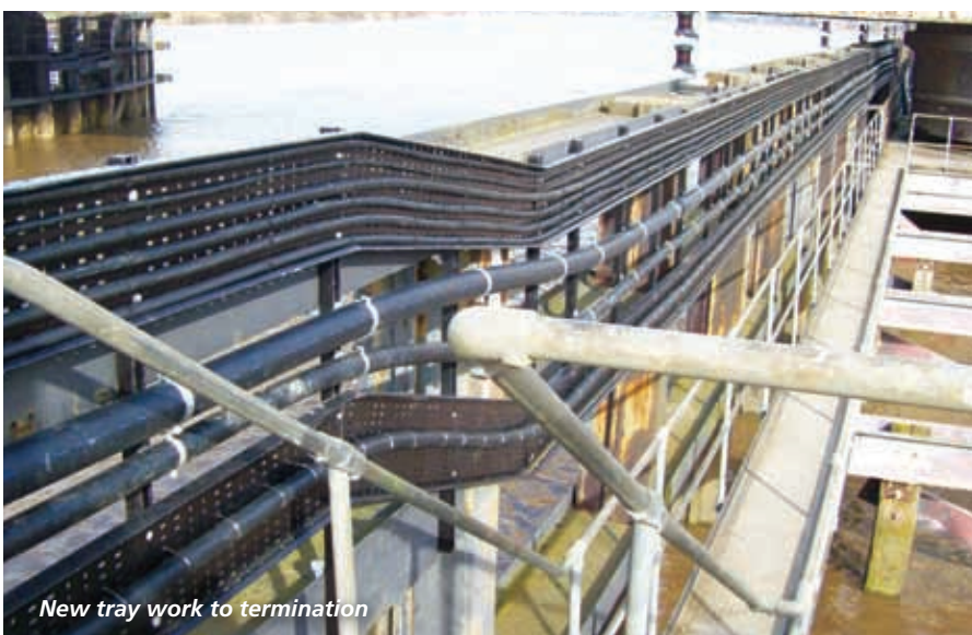
Cables being installed
