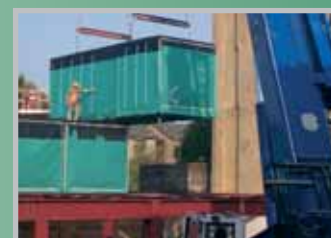
Lowering the module units
