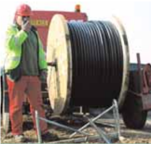
Lutterworth: Cable Pulling
