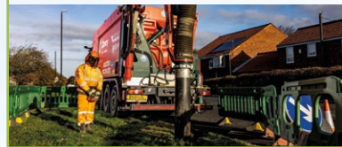
New tools like suction excavators allow us to work more efficiently and sensitively with the environment
