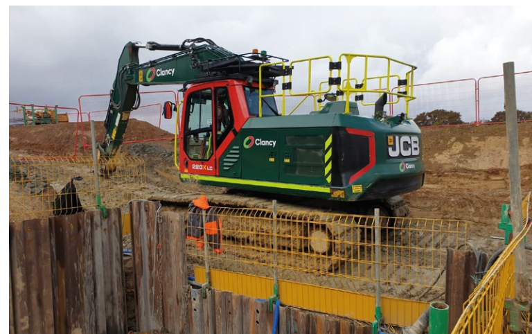
Our excavator at work at the UTX in Faygate
