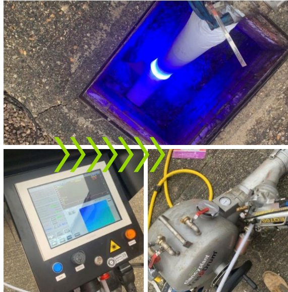
BlueLight site setup and LED light head curing the liner
